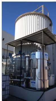
Large-scale WOW demonstration units installed at Saluggia Nuclear Repository (Italy)
